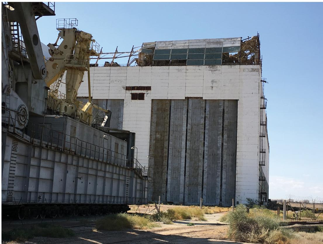
**Figure 3.** The *Buran* assembly building, which collapsed in 2002 with the carrier vehicle in the foreground to the left. Immediately to its left is the Soyuz assembly building. Photo by Cathleen Lewis.
